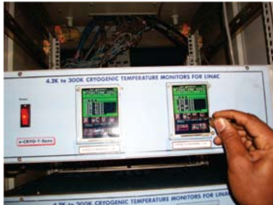
Fig. 10. New cryogenic temperature monitor
