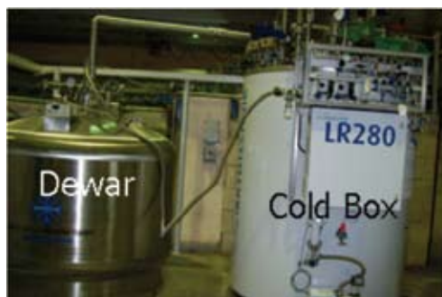
Fig. 3. New Cold Box and 2000L Dewar of New Helium Refrigerator
