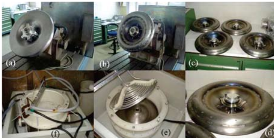
Fig. 3. Clockwise from top left, setups showing the electron beam welding of (a) daisy ribs to the end wall and (b) donut rib to end wall, (c) all four completed end walls, (d) close up view of an end wall (e) electropolishing setup for the end wall, and (f) electropolishing setup for the outer shell.
