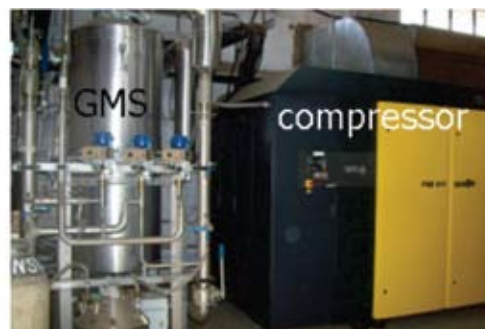
Fig. 4. Compressor and GMS of the New Helium Refrigerator
