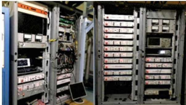
Fig. 3.30 LLRF Electronics Setup in HCI Facility at IUAC
