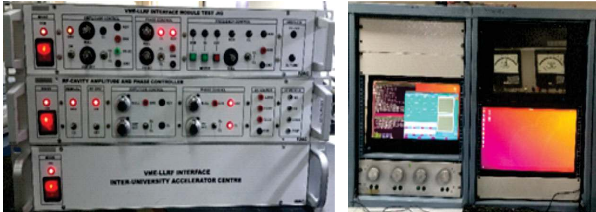
Fig. 3.32 LLRF-VME Interface during Testing and RFQ powered remotely using the Interface
