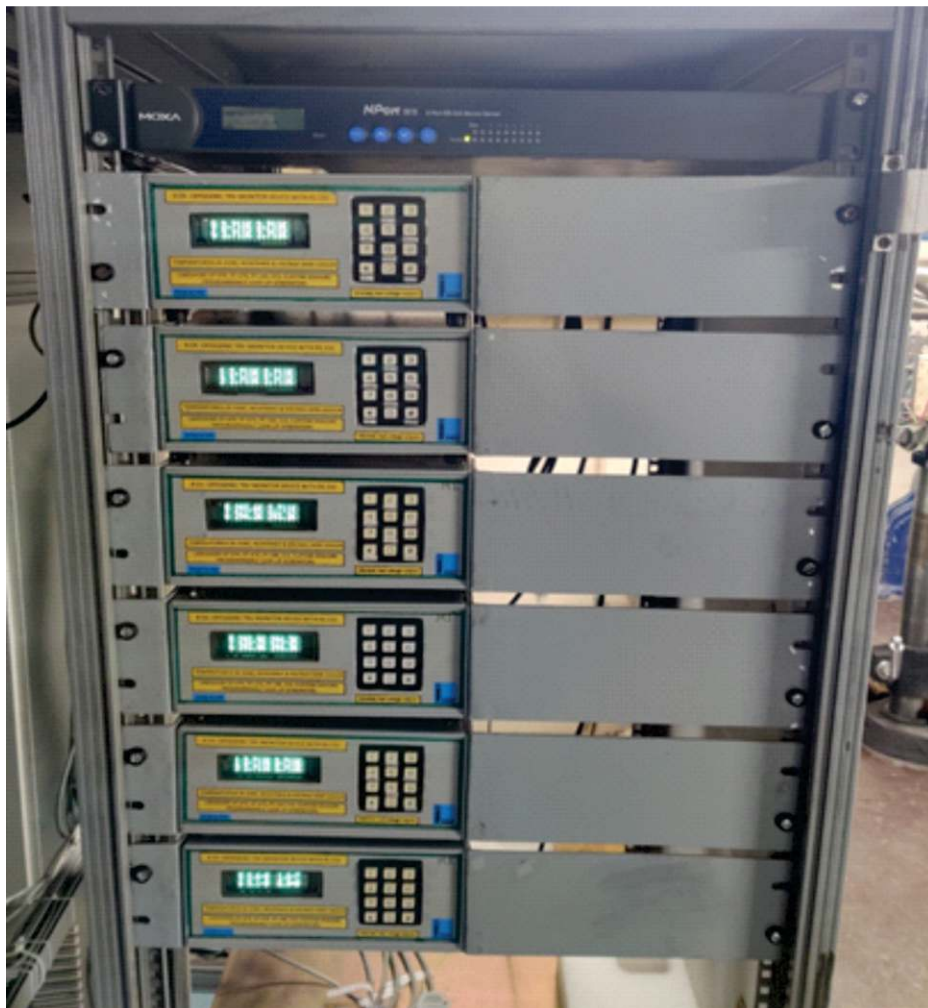
Fig. 3.24 TRV monitors installed in non-radiation area 314 (Old He plant)
