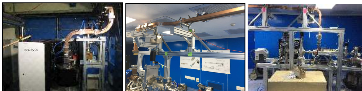
Figure 1. High Power RF system along with waveguide was installed at IUAC
