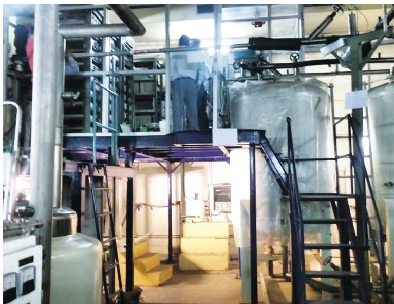
Mezzanine platform for LINAC control room
