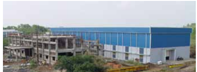
Figure 9 : Building under construction for SCRF infrastructure facilities
