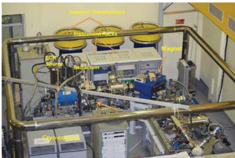
Fig. 3.1.1 HCI High Voltage Platform with ECR and LEBT Components
