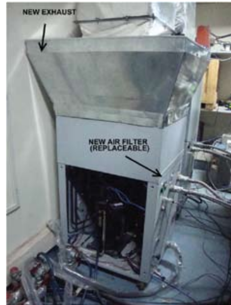
Fig. 2. View of the new extraction cryo-cooler installed
