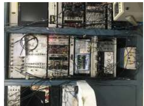
Fig. 1 Pulsing Electronics setup in Control room
