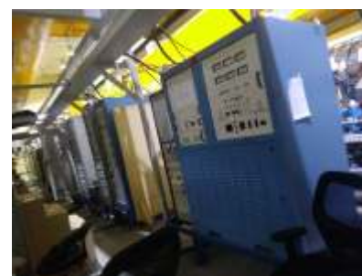
Figure 3: RF Power Supplies
