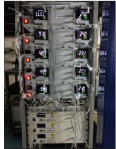
Fig. 1 Newly installed PID switcher unit for the cryogenic control system.
