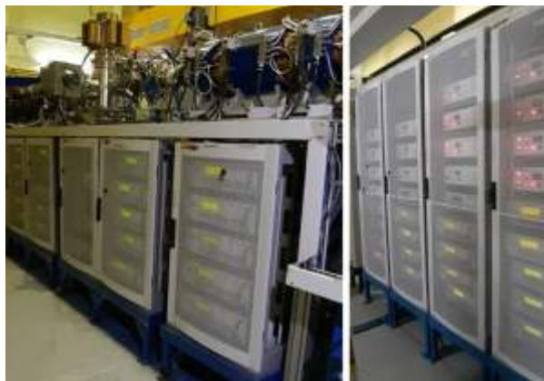
Fig 2: Installation of HCI-BTS magnet power supplies.
