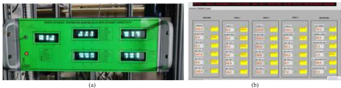
Fig. 4 (a) The newly installed remote temperature monitor and its GUI at the cryogenic control room.
