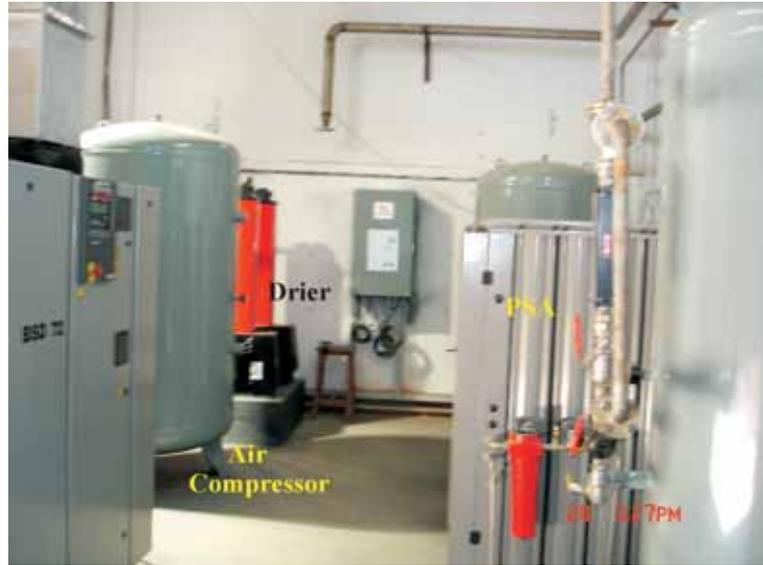
**Fig.3. New PSA system of upgraded LN2 Plant**
